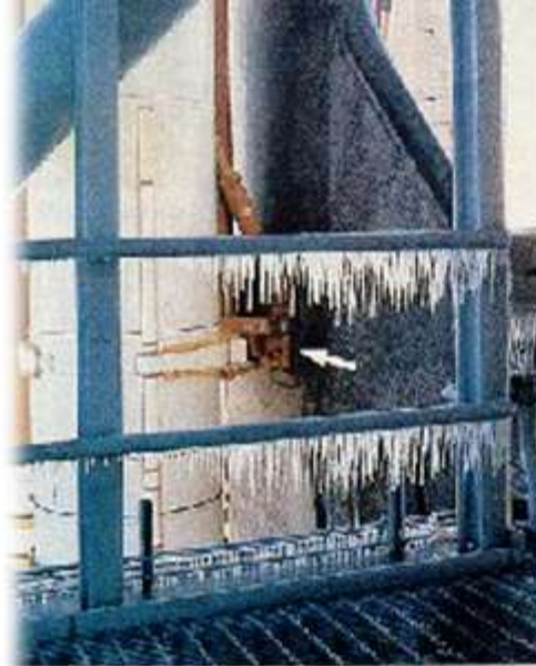
Above, long icicles on a lower rail of the Solid Service Structure frame the launch point where the Orbiter is attached to the external tank. Below, icing was even more extensive on upper levels of the service structure (upper right and below). At right, below, is a ground-to-orbit communications box (not used during launch) that was inoperable by heavy ice.
