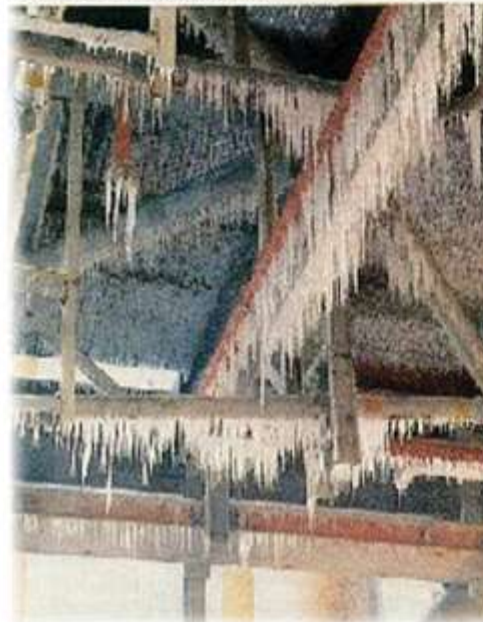
Above, long icicles on a lower rail of the Solid Service Structure frame the launch point where the Orbiter is attached to the external tank. Below, icing was even more extensive on upper levels of the service structure (upper right and below). At right, below, is a ground-to-orbit communications box (not used during launch) that was inoperable by heavy ice.
